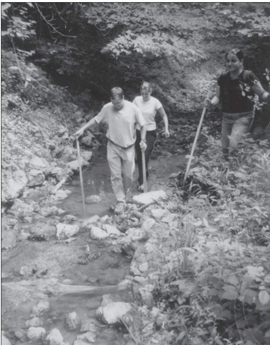
Figure 6. Ravine Park Ravine 13 years after construction with fully established vegetation. Sand and silt from the eroding upstream section of the ravine has filled the interstices of the stone in the ravine bed. Note 12-inch to 24-inch stones forming natural weir (check dam).
