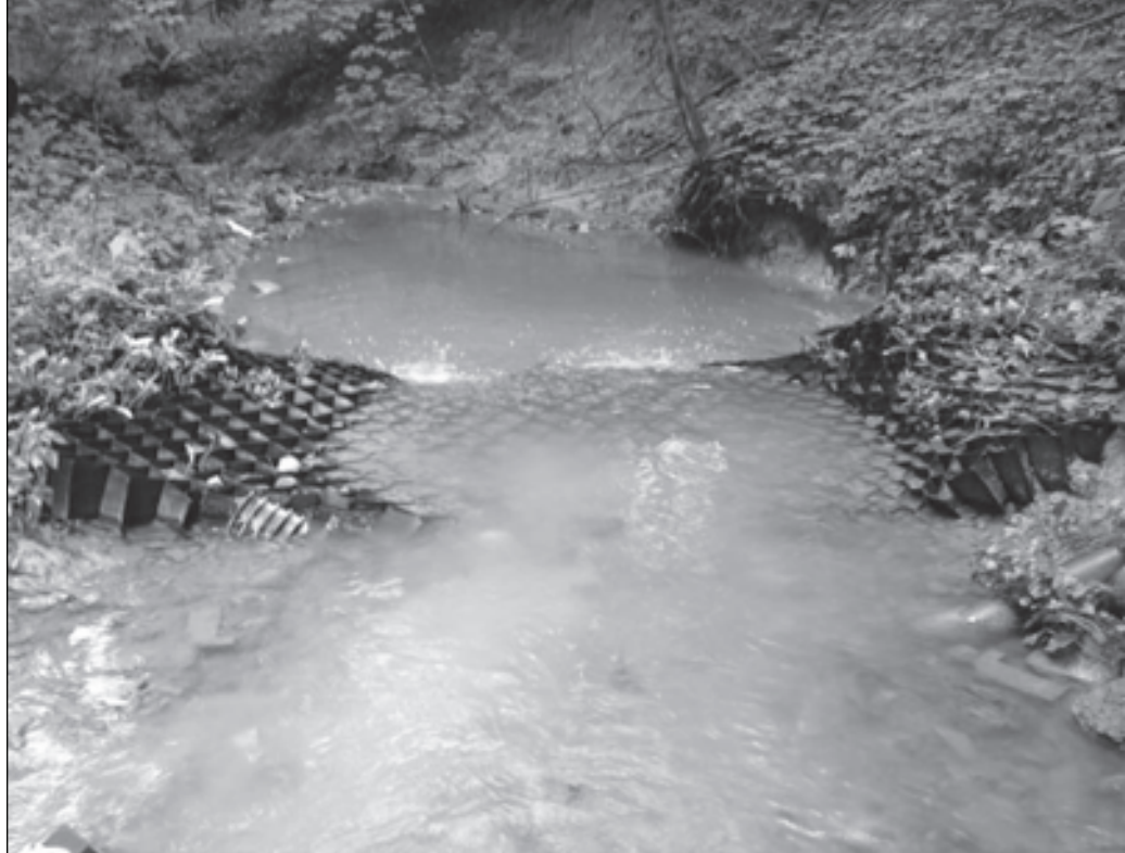
Figure 20. Geoweb armor intact in 2007. Note loss of natural streambed armor and fill-stone.
