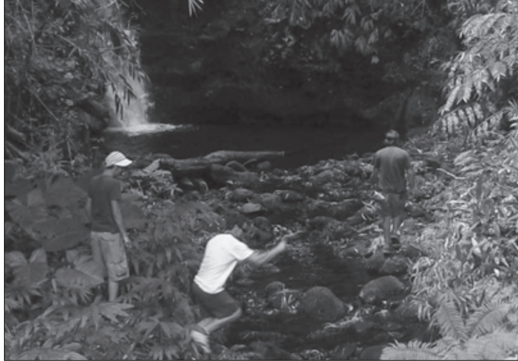
Figure 14. A plunge pool protected by the proper size boulders makes a more natural energy dissipator at a stormwater outfall than one protected by gabions.
