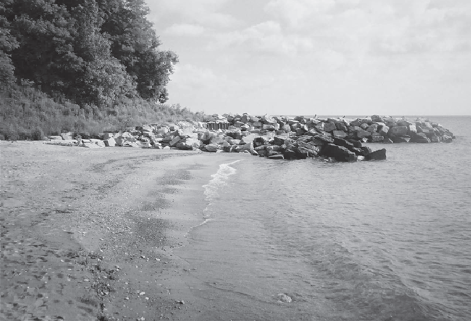
Figure 7. Newly constructed pocket beach at mouth of Ravine Park Ravine, Lake Bluff (2007 photo). Note well established vegetation on bluff stabilized in 1990. Periodic air photo surveys show the beach to be stable with no negative impacts on adjacent beaches.
