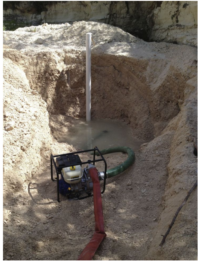
Photo 3. Anse-à-Galets Pump Test Configuration
